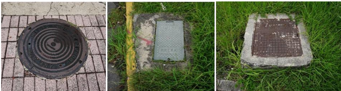
Photo 18: Cast Iron MH cover marked PUERTO RICO TELEPHONE COMPANY (left); subterranean utilities access boxes, marked PREPA (center), and DTOP (right)
