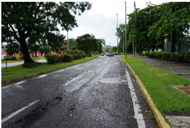
Photo 14: Segment of PR-2R
