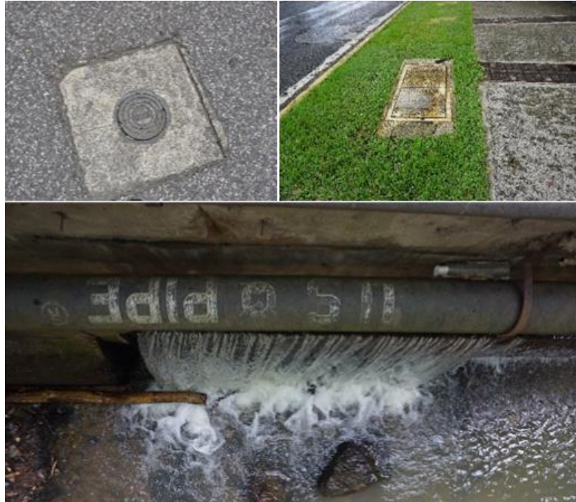
Photo 17: Left: sewer access; right: unidentified MH cover
