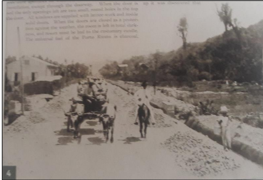
Figure 15: Road under construction, photo by Walter Townsend, 1898 (from Sepúlveda 2004, 3: 256)
