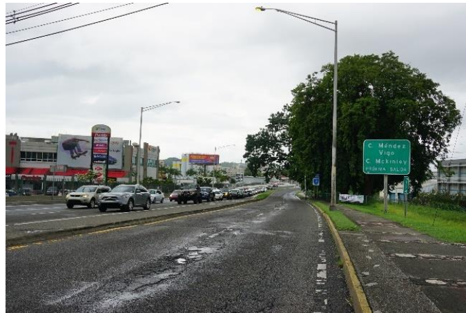
Photo 15: View of PR-2 towards project end, looking south
