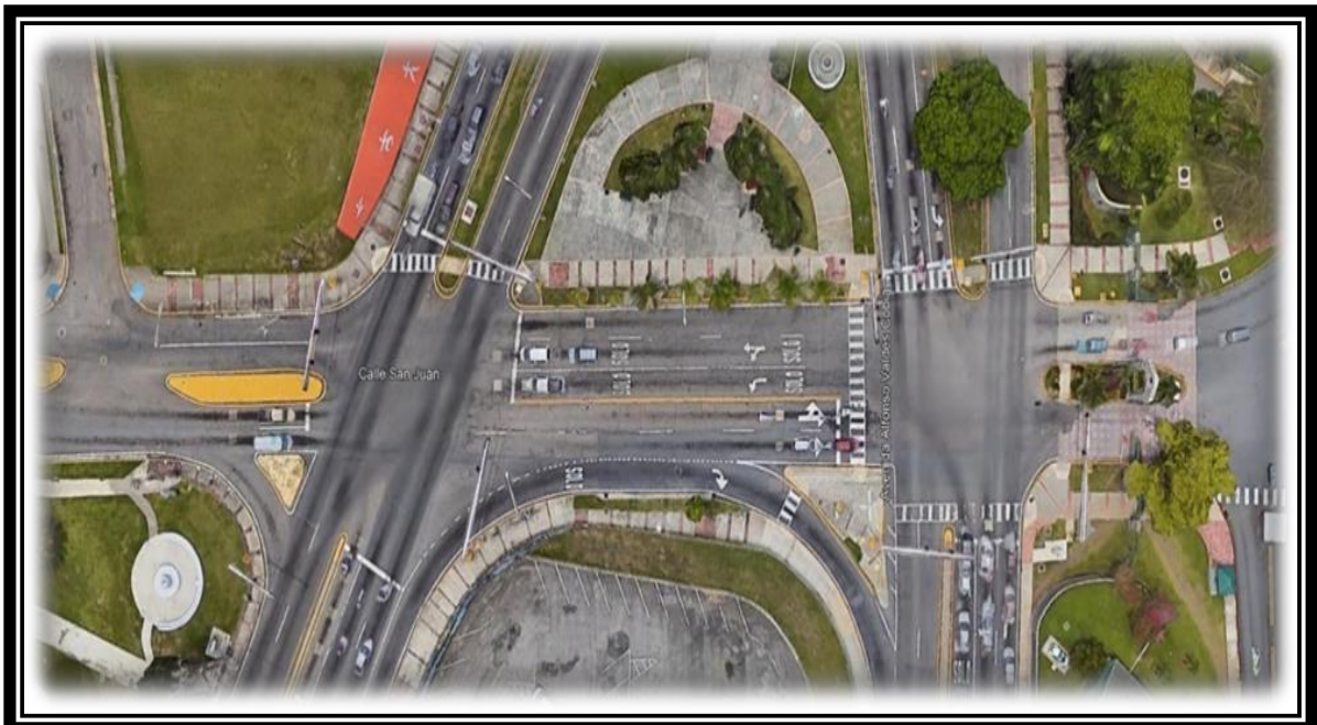
Figure M – Highway PR-2 with San Juan Street and PR-2R (RUM Entrance).
